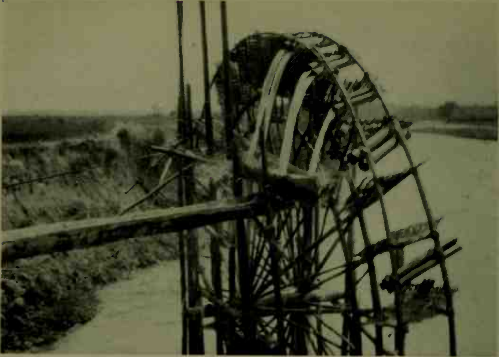
Lifting in sections of bamboo set at a slight angle the water of the streams that turn them, the home-made water-wheels of southern China pour it into crude troughs that carry it off to the fields
